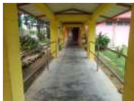
e) Corridor with handrails
