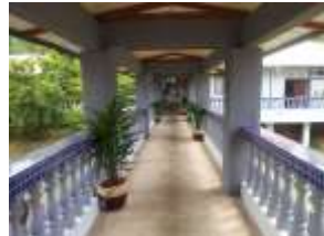
c) Bridge that link to Admin Block
