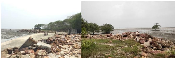
Figure 3: Images of Pantai Jeram and its current view in 2020 (Source: Author)
