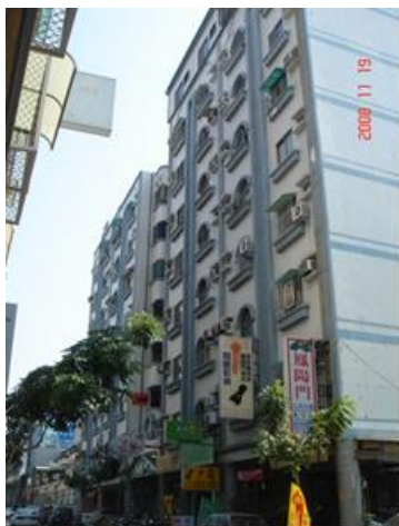
Fig. 6. Facade of the test building assessment framework
